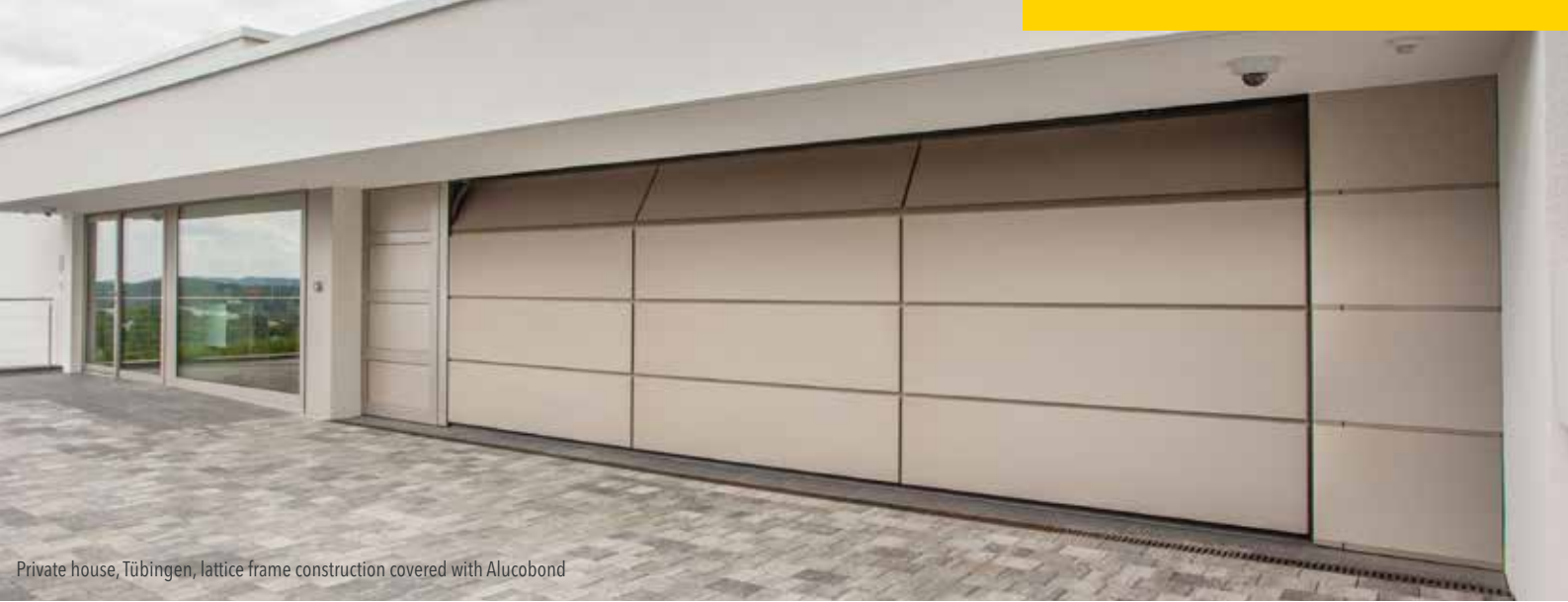
Private house Bissingen, lattice frame construction covered with aluminum composite
