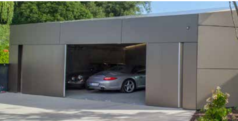
Private house, Tübingen, lattice frame construction covered with Alucobond
